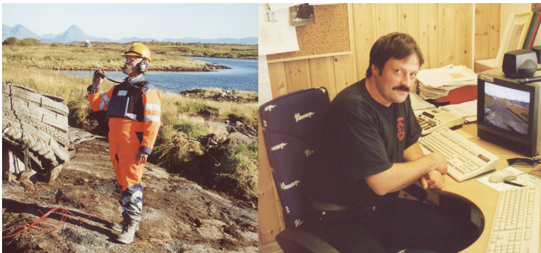
Figure 4 A remote inspection situation from road construction where the field worker gets assistance from an expert in his office
